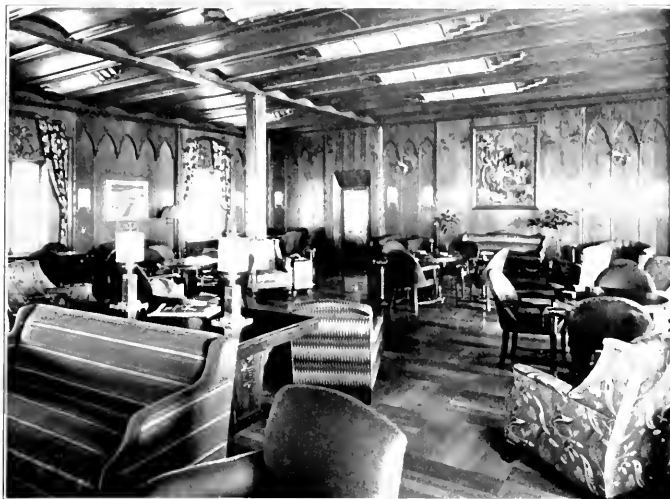
The smoking room of the Dollar liners is finished in dark Buntinga paneling. Adequate illumination is secured by the use of unusually large ceiling fixtures in cylindrical form nested in the coved ceiling.
